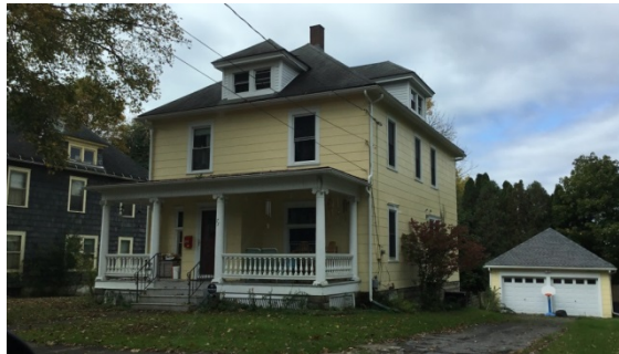
71 Chapin Street. Owner Occupied Housing Rehab project completed in 2017
