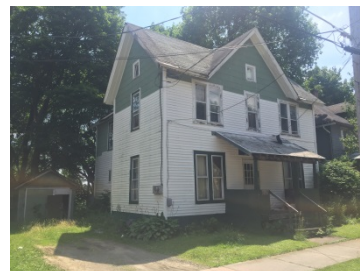
2017 Demolition Projects; 120 Bush, 111 Barrows, 64 Grant.
