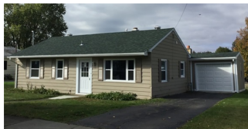
320 Delaware Street. Completed by CHRIC in 2017 ($37,044.00 Committed from Jamestown). Recently sold to new homeowners
