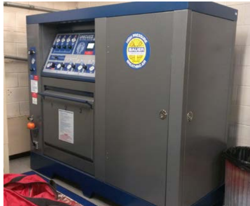
New SCBA Compressor Fill Station
