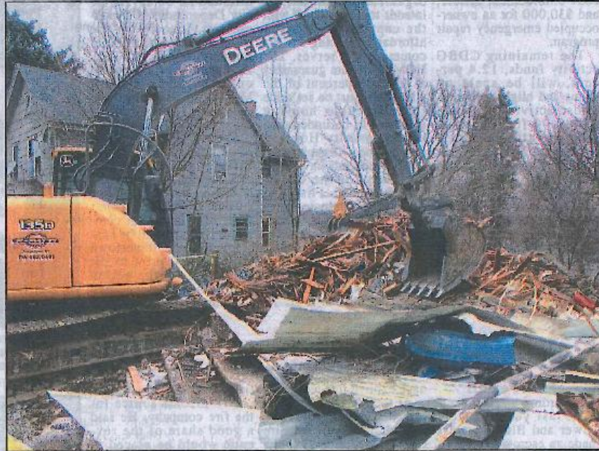
Construction crews tearing down a condemned house on Willard Street in December 2014. City officials use U.S. Department of Housing and Urban Development funding to demolish condemned houses.
